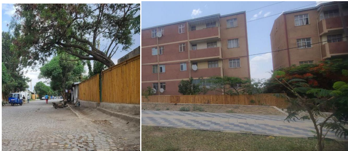
Figure 23: bamboo fence around harambe university Figure 24: goro condominium fence
