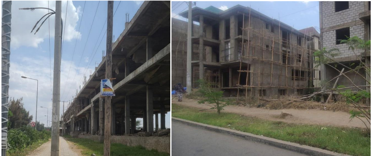
Figure 21: frontage under construction around adama tractor factory Figure 22: kebele 11
