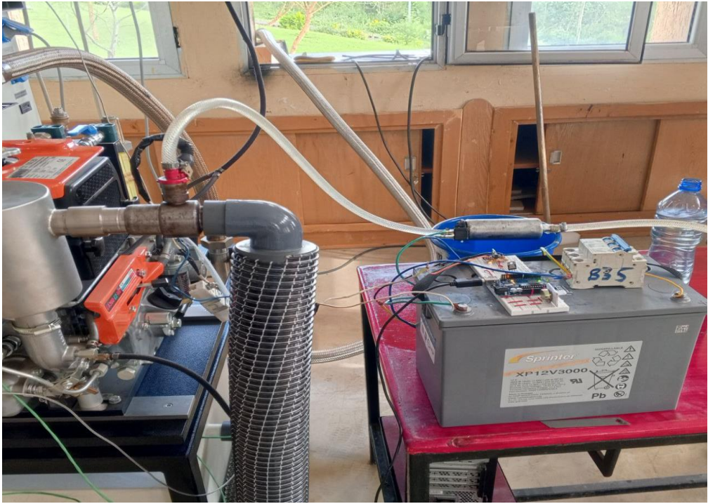
Port injection system setup
