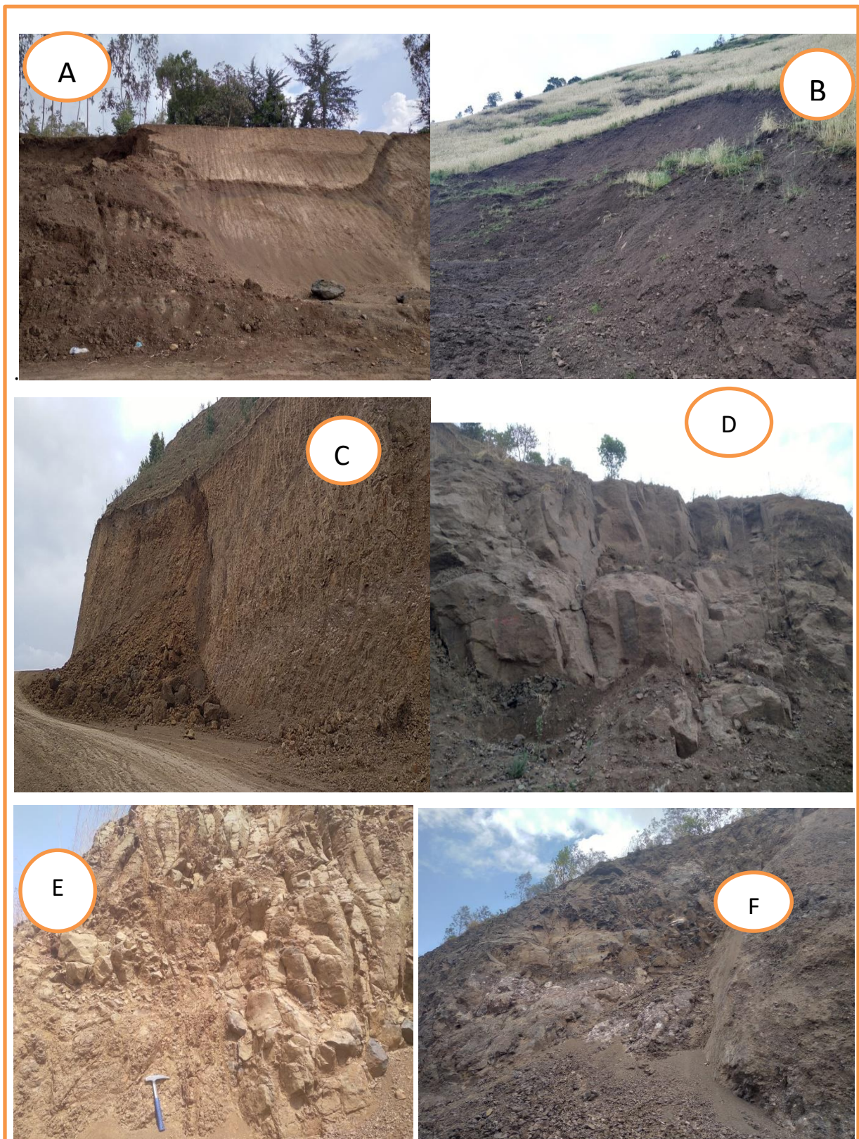
Figure 3.1 Critical sections of soil and rock slopes A) soil slope section six, B) soil slope section three slope C) highly weathered basalt, d) ignimbrite E) slightly weathred basalt F) moderately to highly weathred basalt.
