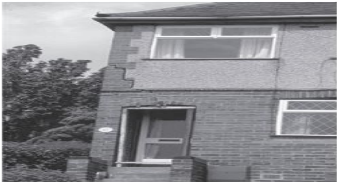
Figure 8: Structural damage to house caused by ‘end lift’ (Lee D Jones ,2012).
