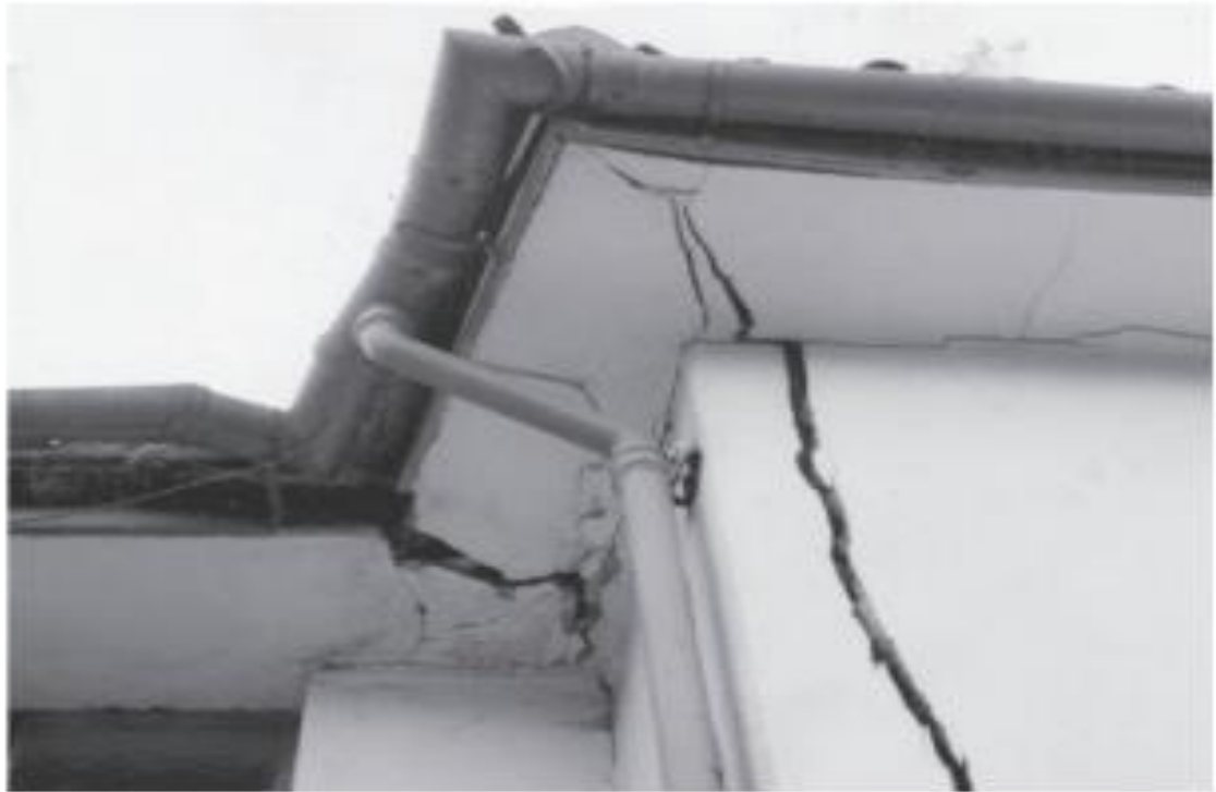
Figure 8: Structural damage to house caused by ‘end lift’ (Lee D Jones ,2012).
