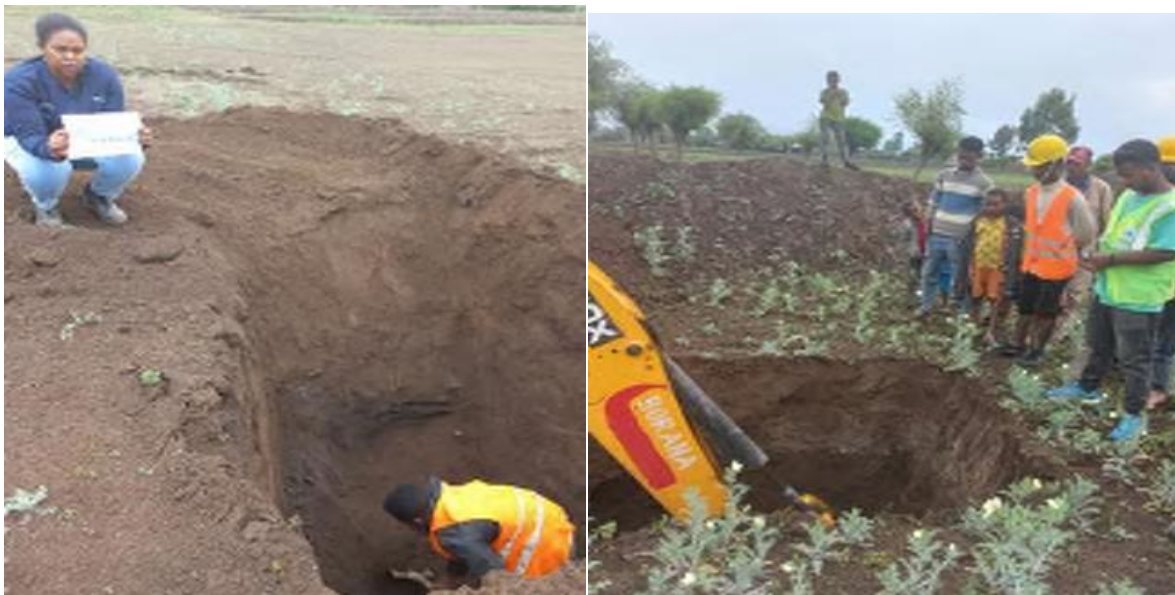
Chainage at 11+100 Centre
