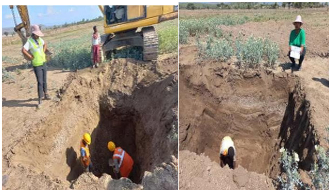
Chainage at 11+900 LHS
