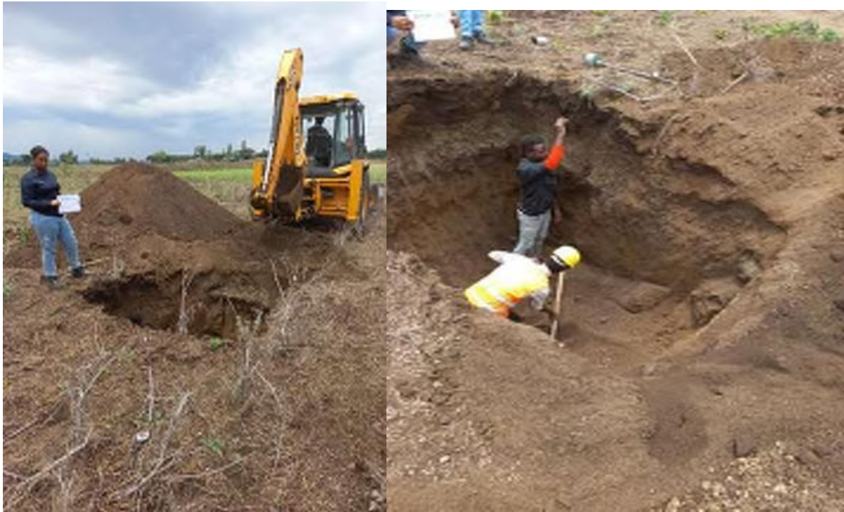
Chainage at 10+900 LHS
