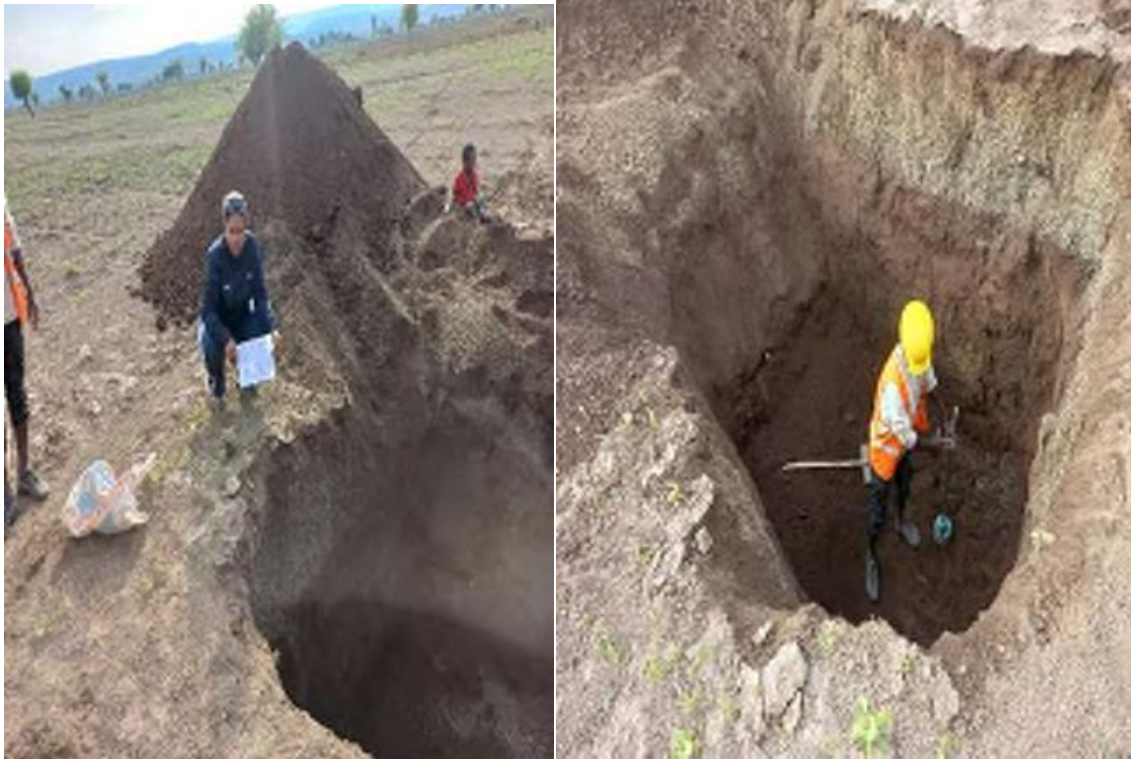
Chainage at 10+100 RHS
