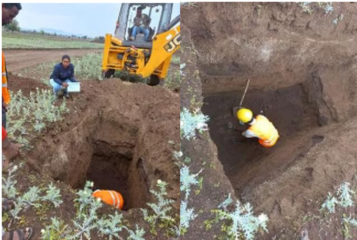
Chainage at 11+300 RHS
