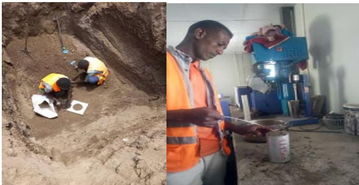
Chainage at 11+500 Centre
