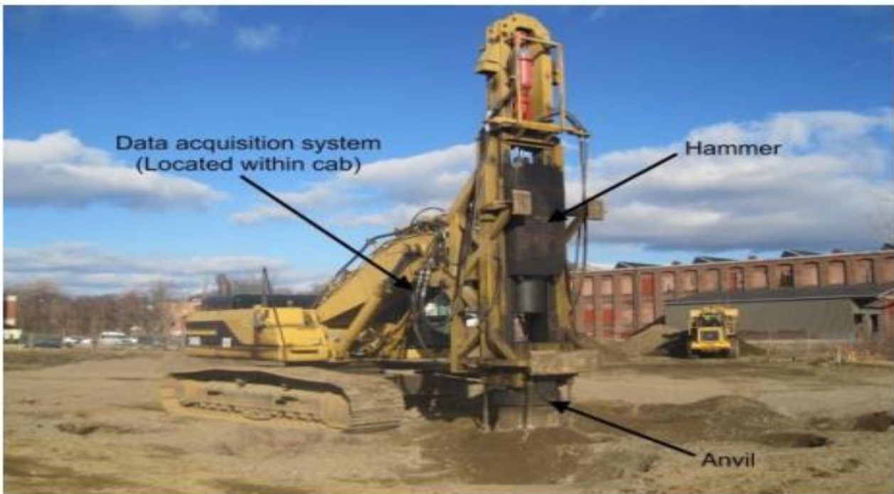
Figure 2.10: A Typical RIC Unit (Becker, 2011)
