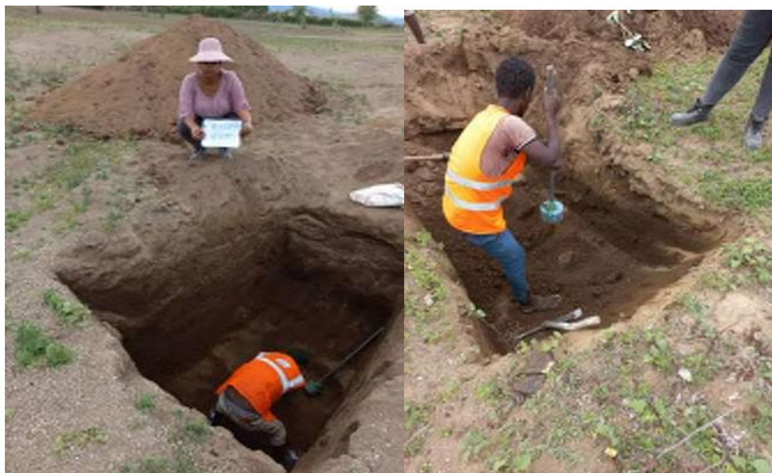
Chainage at 8+100 Centre
