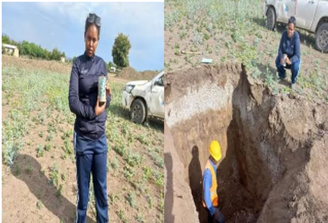
Chainage at 10+500 Centre
