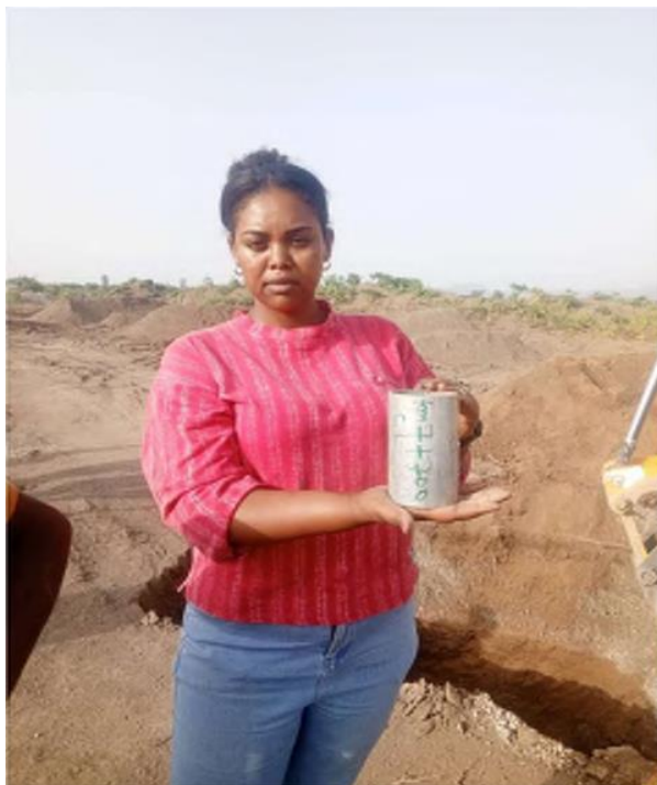
Chainage at 7+700 Center
