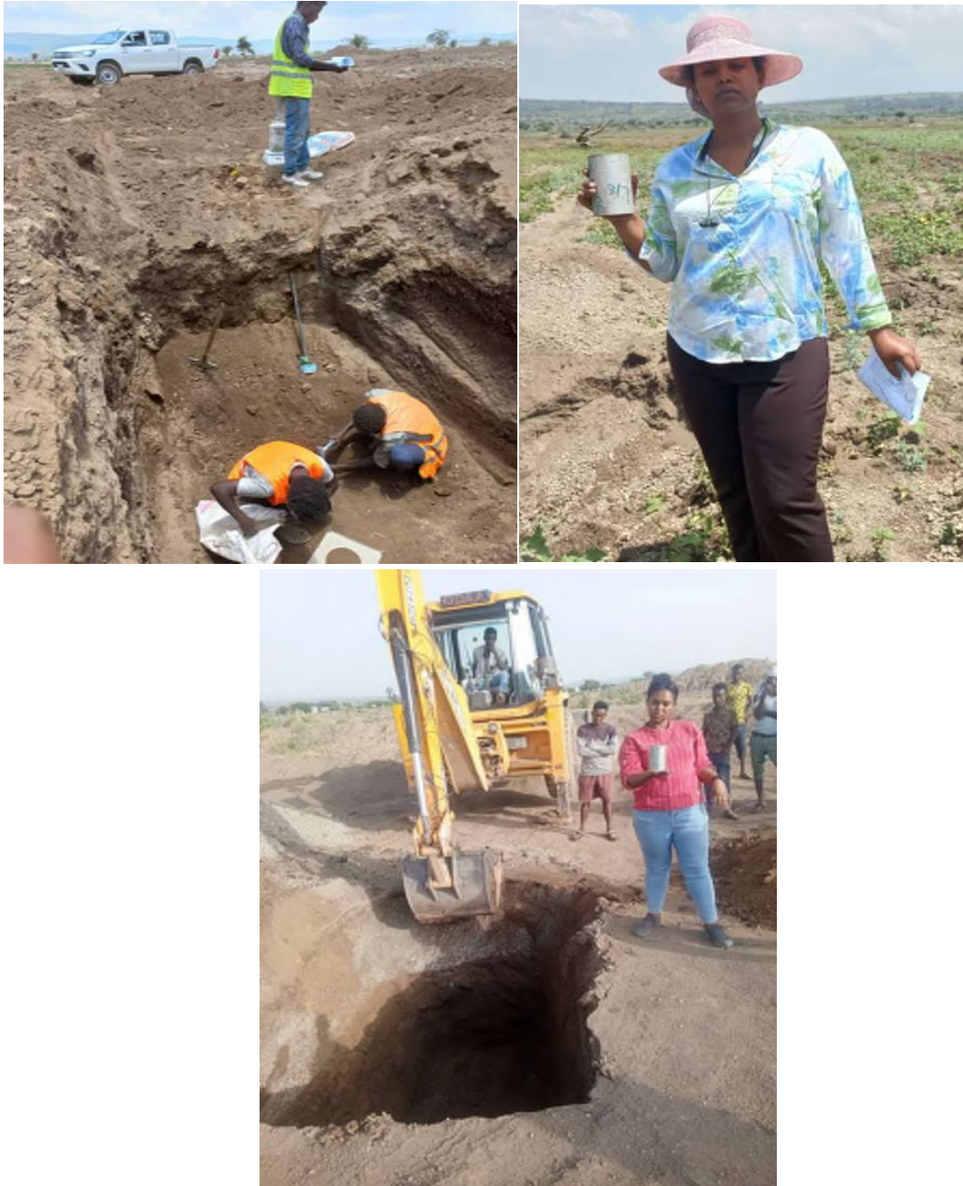
Chainage at 7+500 RHS
