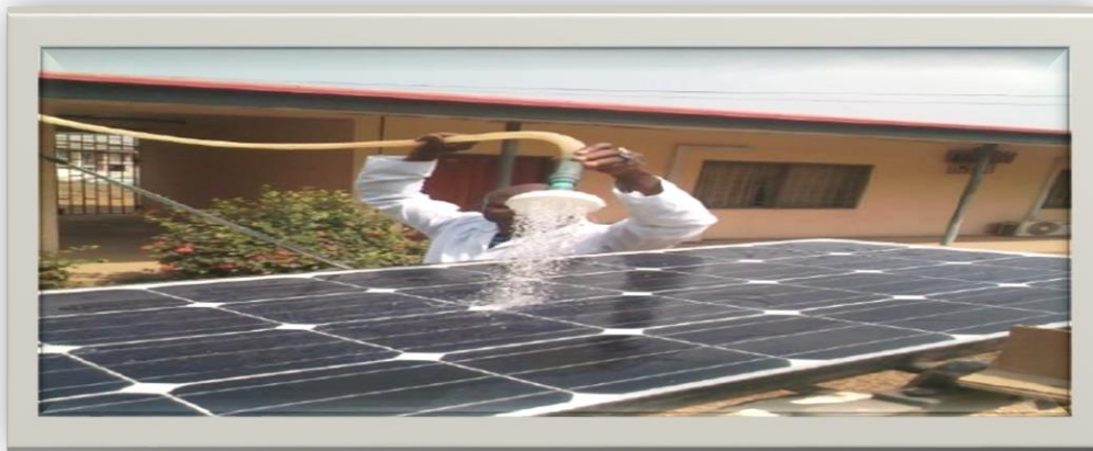
Figure: 2. 4 Photovoltaic modules cooled with water cooling system (Ale and Rotipin, 2019)
