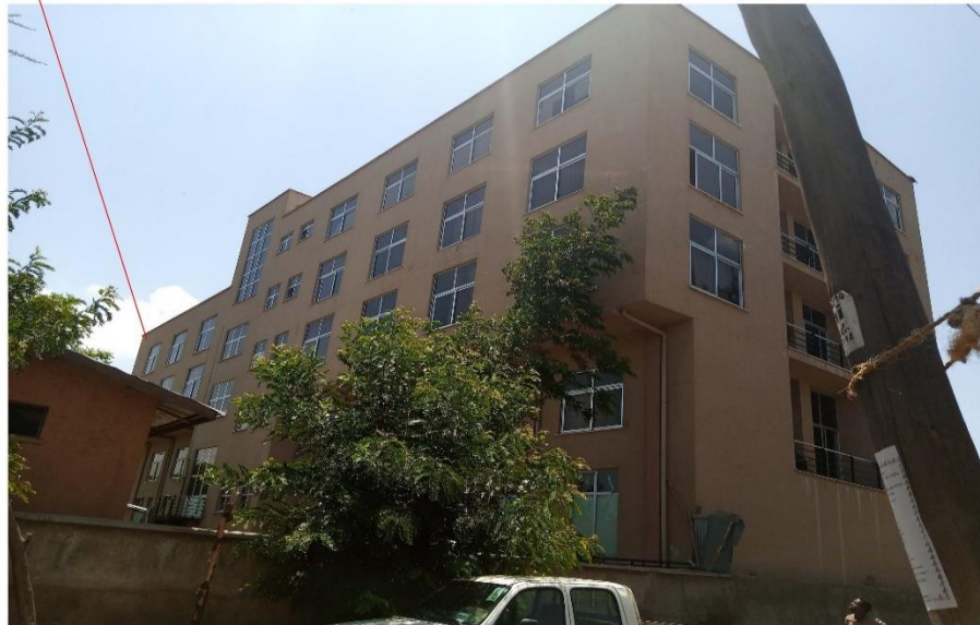
Figure 9: A building with a concrete roof
