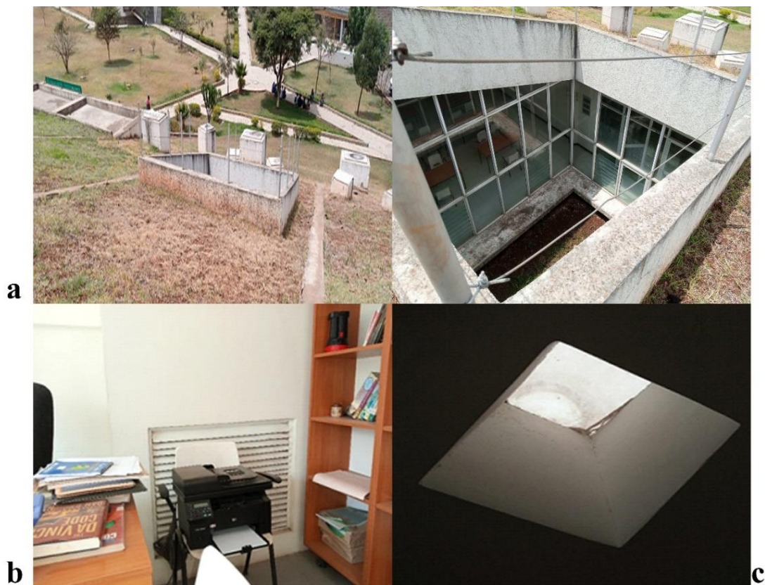
Figure 14: Henk de Pagter Library Building a) Open Down and Duct boxes b) Vent duct inside the office c) skylight
