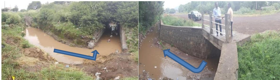
FIGURE 4.11: Critical Outlets condition of Ziquala Catchment at lower reaches. (Source: field surveying).
