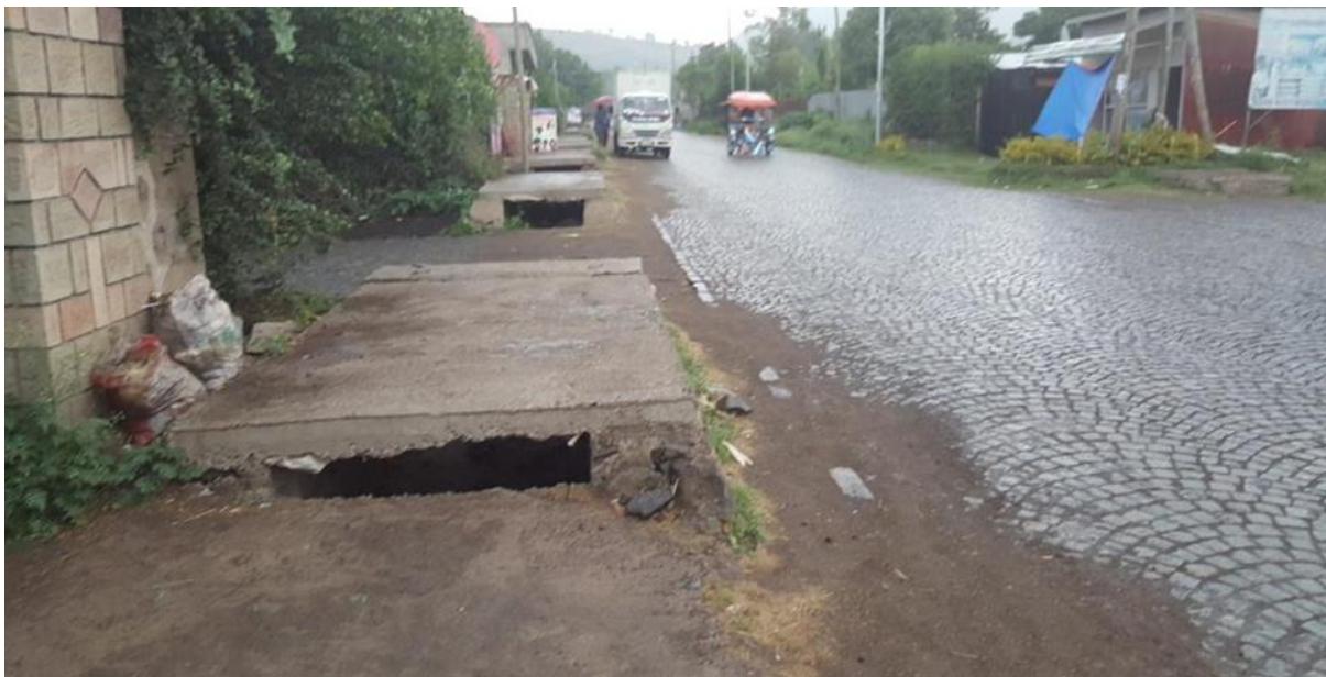
FIGURE 4. 3: Drainage & Road Infrastructure Development (Source: field surveying)
