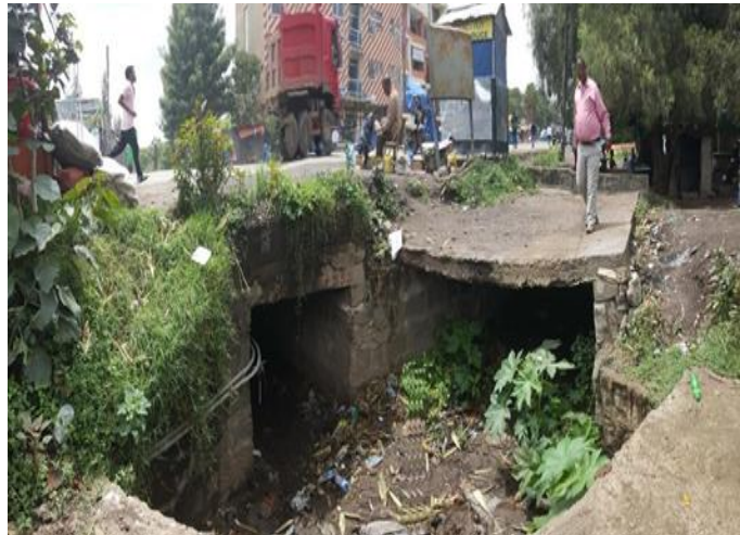
The drainage line in front of bus station seriously blocked with silt-up of mud and waste
