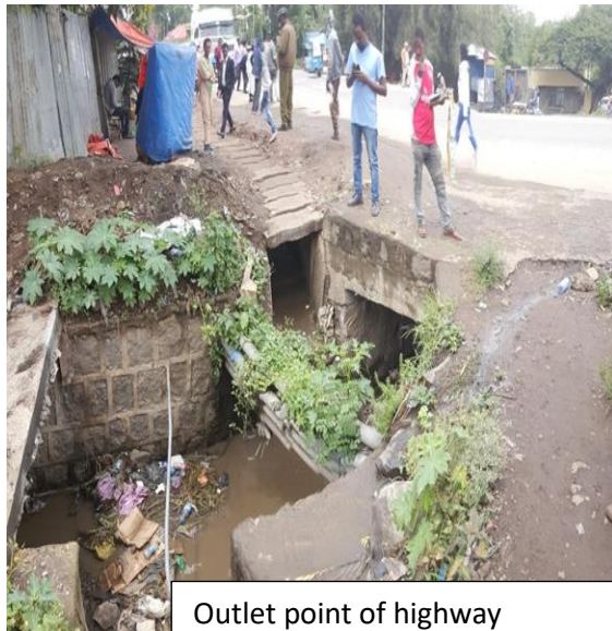
The drainage line in front of bus station seriously blocked with silt-up of mud and waste
