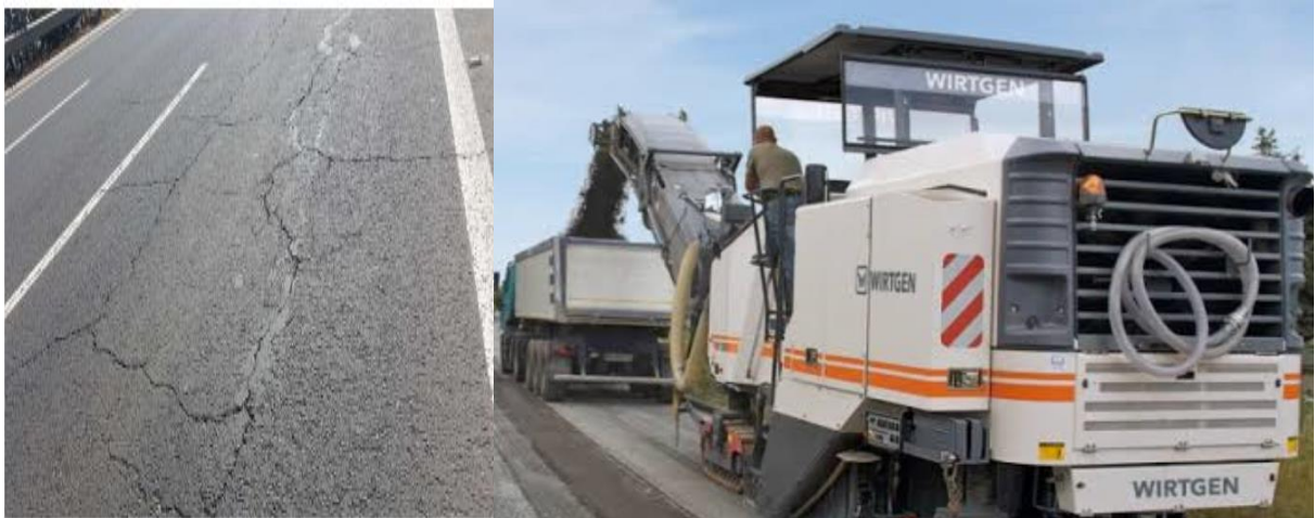
Figure 3-1: Cracked surface and Milling machine extracting the RAP near IT park.
