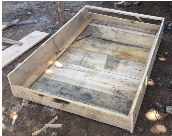
Figure 3.14: Collector box construction
