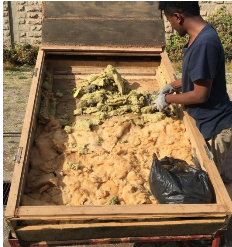
Figure 3.16: Collector fiber glass insulation insertion
