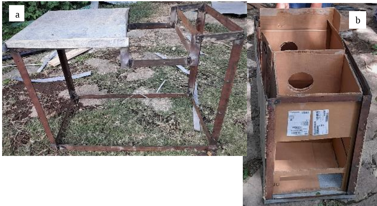
Figure 5.10 Manufacturing process of 2-pot BCS pattern a) preparing the edge supports and b) preparation of the internal pattern
