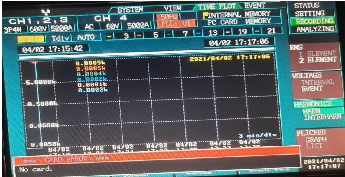
Figure A.7 Phase1 Current Harmonics reading on the Harmonics Analyzer on load side of VFD drive
