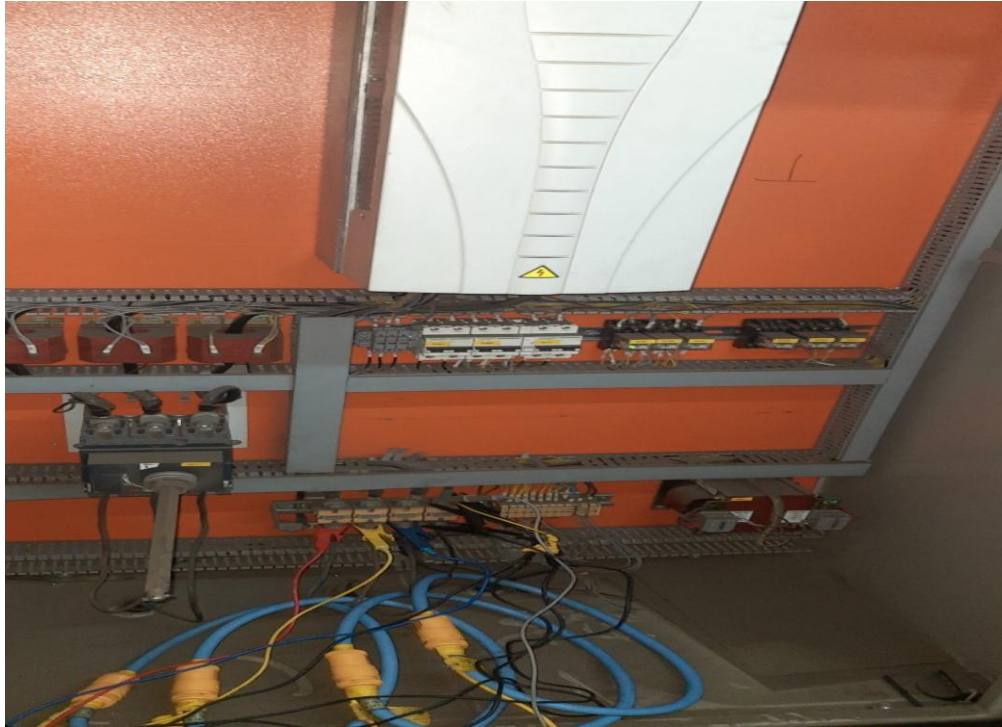
Figure A.5 Connection of Harmonics Analyzer on load side of VFD drive
