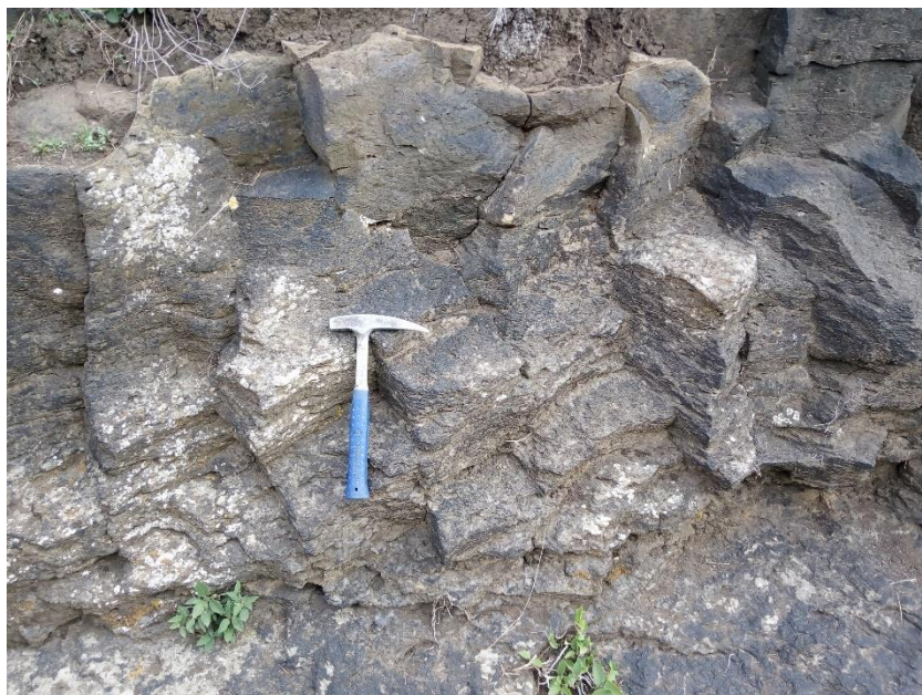
Figure 4. 5. Joints and their representative description of the dam site (joint sets at the right abutment).
