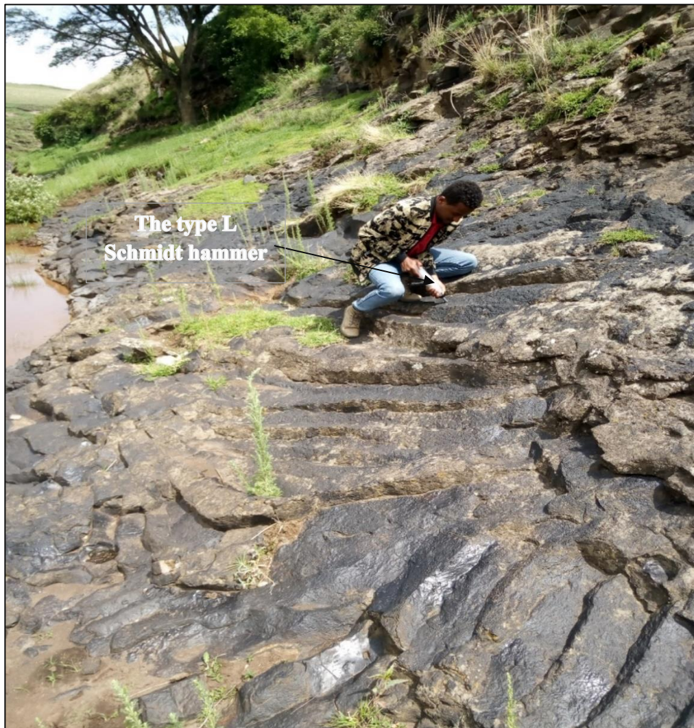
Figure 3. 1. The type L Schmidt hammer test on the left abutment ignimbrite rock mass.
