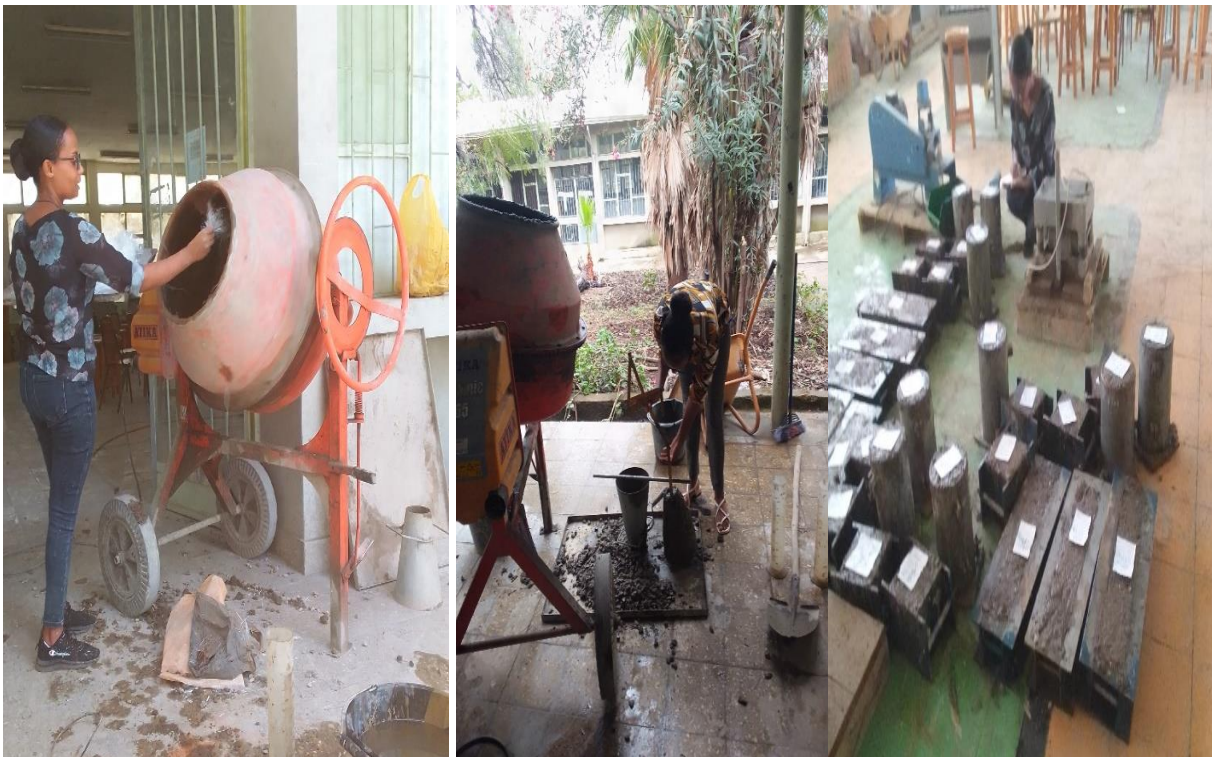
Appendix E4: Pictures captured during casting of concrete.
