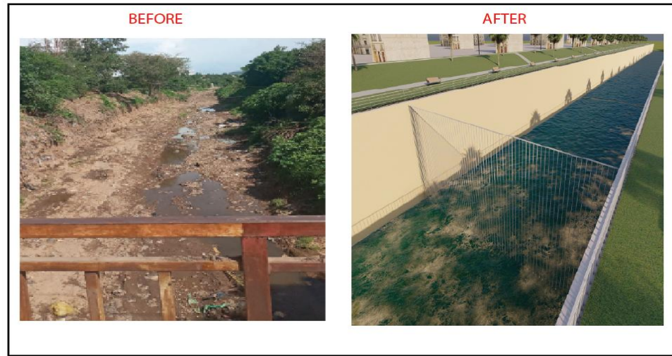
Figure 33 Before and after the design of solid wastes and other filtering fences
