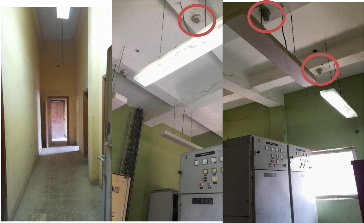
FIGURE 1. 1. Overhead picture of a smoke detector on the ground floor
