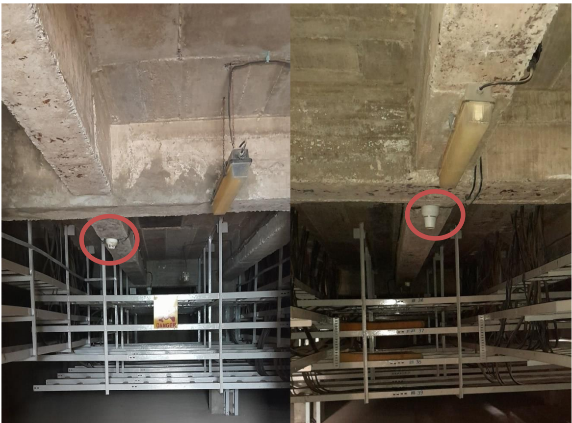
FIGURE 1. 1. Overhead picture of a smoke detector on the ground floor
