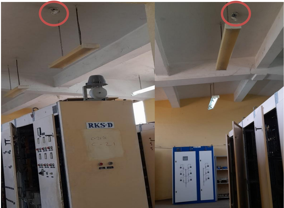
FIGURE 1.3. Overhead picture of a smoke detector on the Second Floor
