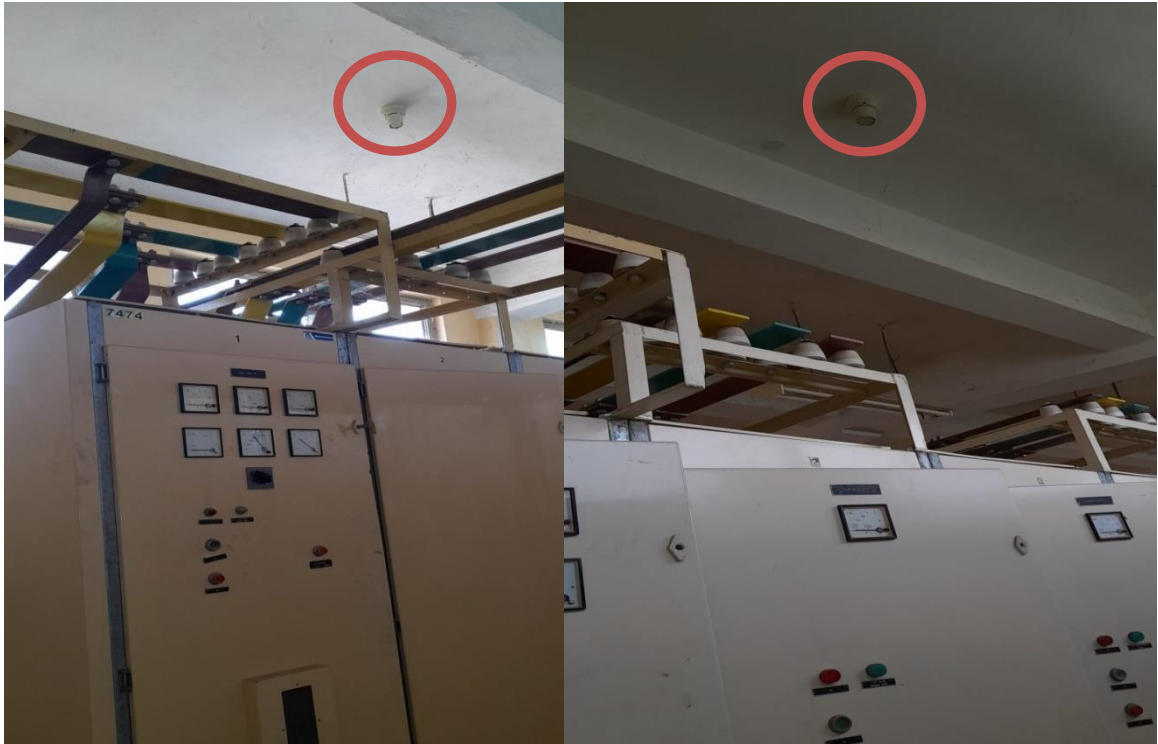
FIGURE 1.3. Overhead picture of a smoke detector on the Second Floor
