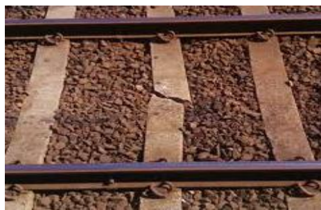
Figure 1.2. Sleeper braking of old railway found at Dire Dawa
