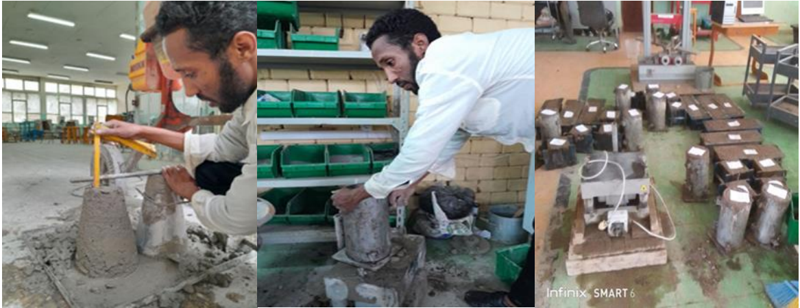
C1.3: Pictures captured during casting of concrete.
