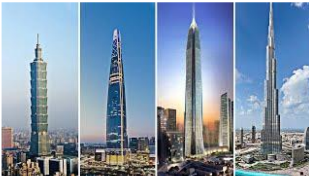
Figure 1-1: Example of the highest-glazed high-rise buildings in the world
