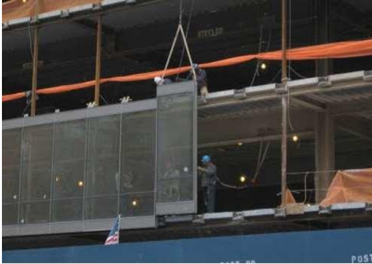
Figure 2-4: Unitized or modular built curtain wall system (Orlowski et al., 2018)
