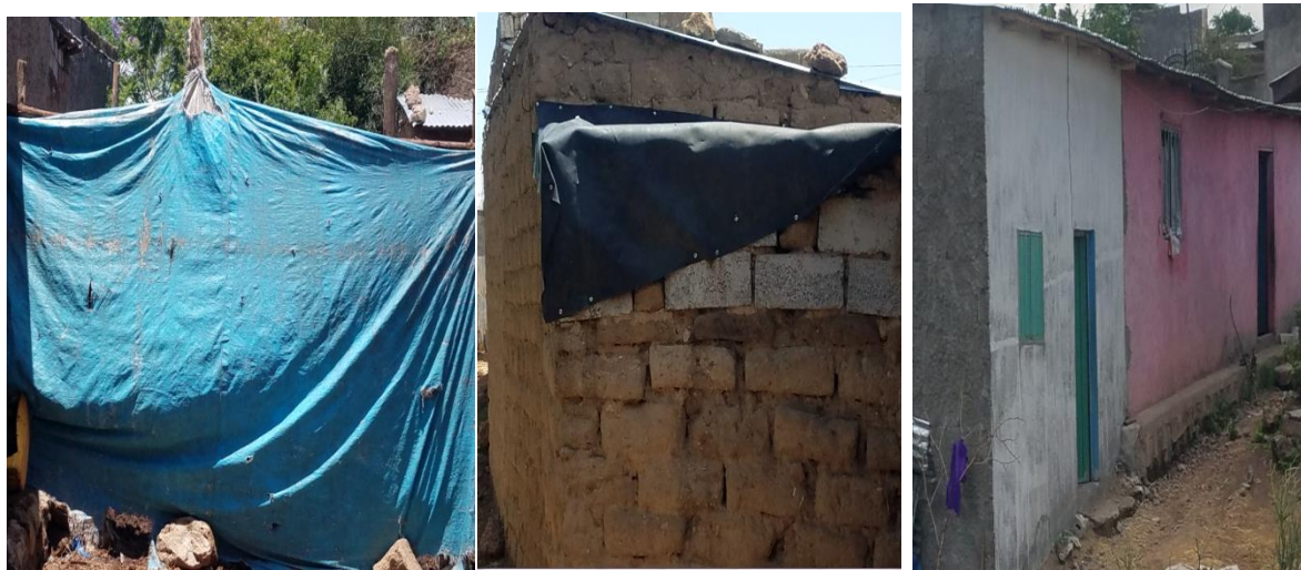
Figure 4.1. Housing construction material and their durability status
