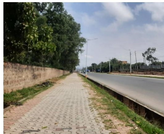
Figure 2.3: Fence building material (masonry work)
