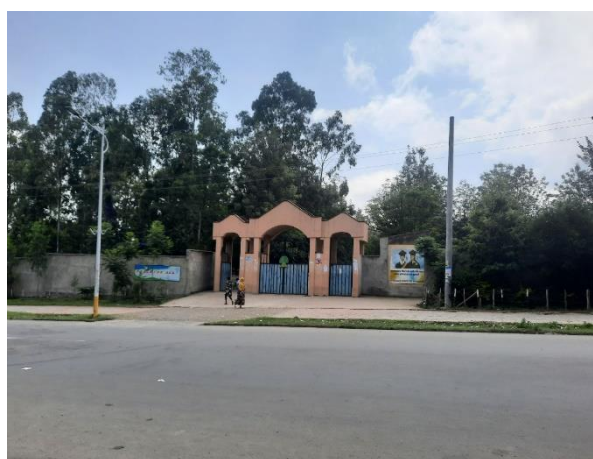
Figure 4.6: Preparatory school (North-East direction)
