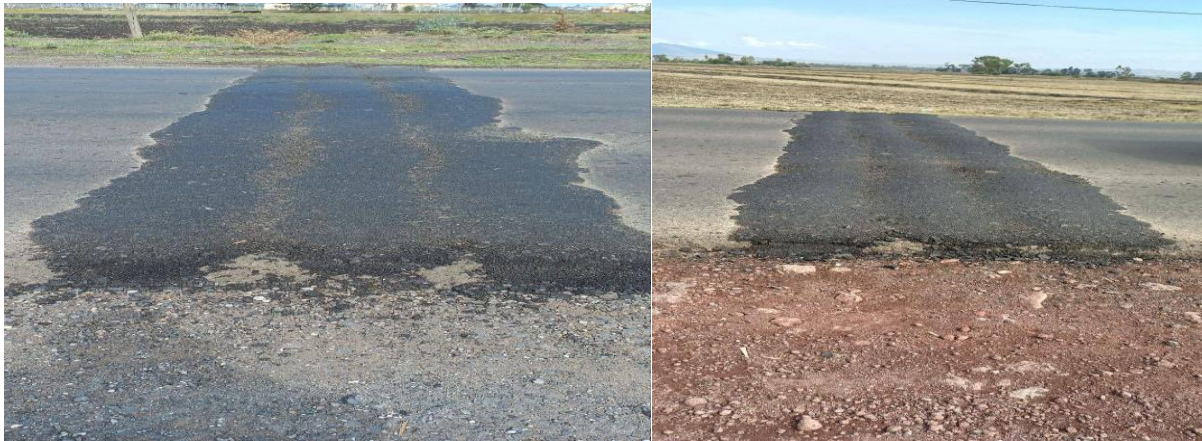
Figure 4.14. Installed road barriers at Burayu Subcities
