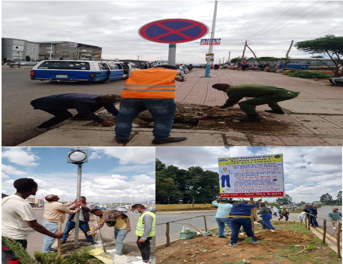
Figure 4.15. The installation of different road safety signs in Burayu Subcity
