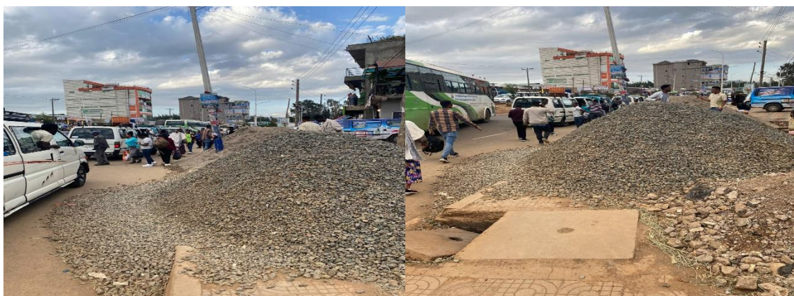
Figure 4.12. Dumping of construction materials on the road at Burayu Subcity
