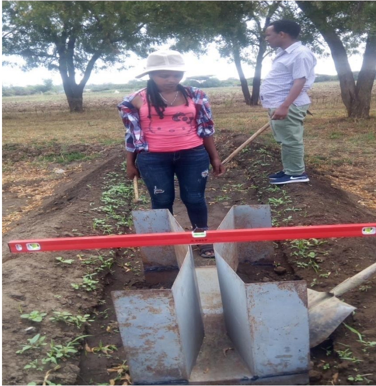
Figure 4 Parshall flume installation
