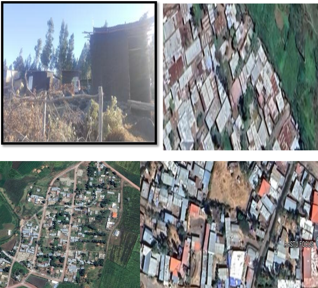
Figure 4.4 Construction materials of the houses and condition
