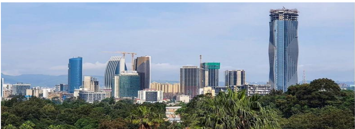
Figure 2.1 :High rise buildings in Addis Ababa, Ethiopia
