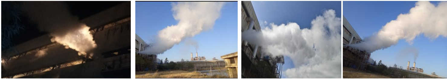
Figure 4.2 image of an excess amount of steam loss to atmosphere in WSSF
