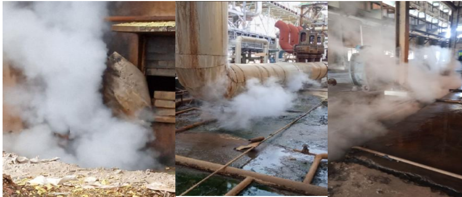
Figure 4.7 Steam loss through leakage at different unit operations of WSSF
