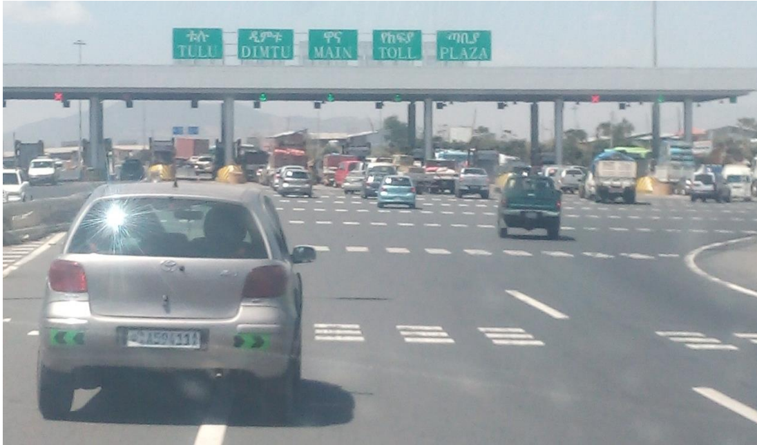
Figure 2.3. Tulu Dimtu main toll plaza
