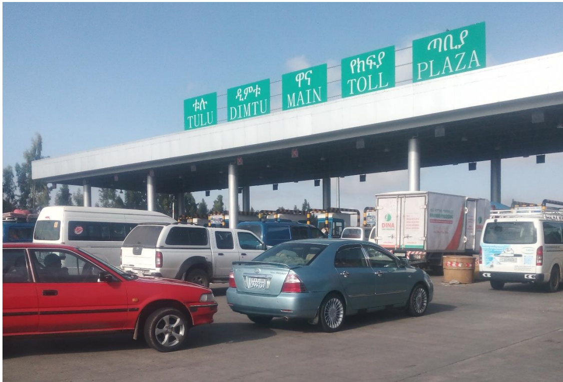
Figure 4.2. Tulu Dimtu main toll plaza, Addis Abeba
