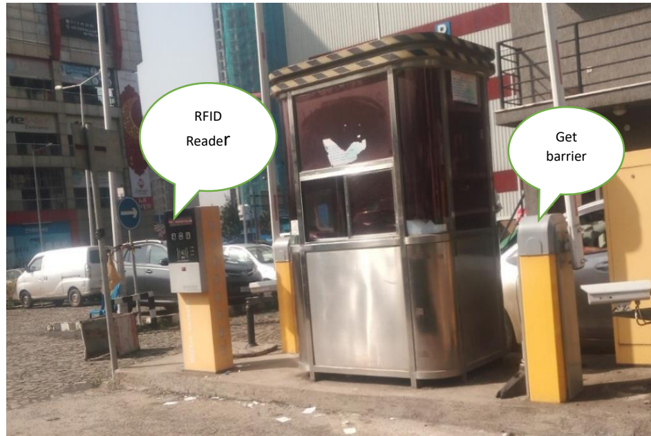
Figure 3.13. RFID based automatic vehicle detection
