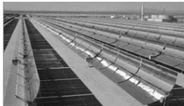
Figure 2.13. Line focusing parabolic trough collector ,the solar parabolic trough mirror (Algeria)
