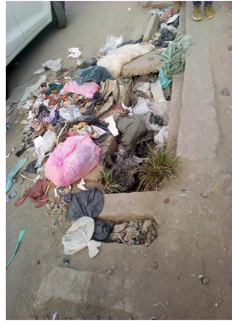
Figure 4.5 The improper disposal of liquid and solid waste into the drainage system.
