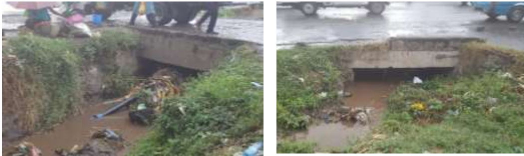
Figure 4.4.3. Existing storm drainage facilities
