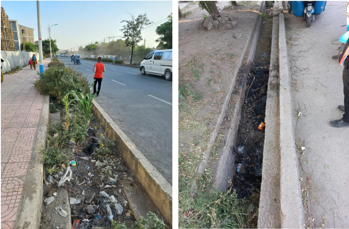
FIGURE 12: ILLUSTRATION OF DRAINAGES BEING USED AS BURNING AREA
