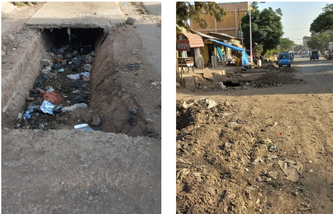
FIGURE 19: SITE A CURRENT DRAINAGES STATUS
