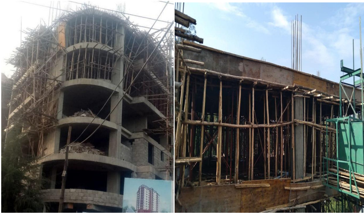
(a) Conventional (wooden) formwork
