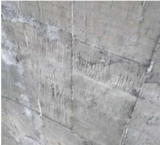
(a) Wooden formwork concrete surface
