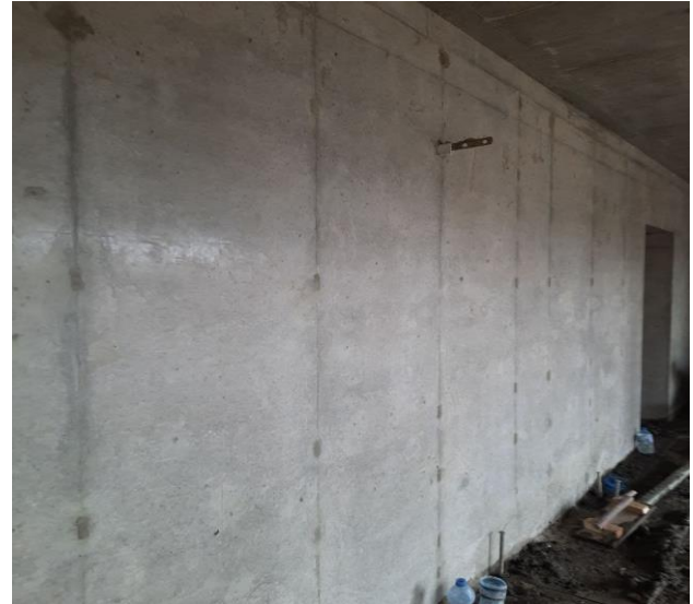
(b) Kumkang aluminum concrete surface
