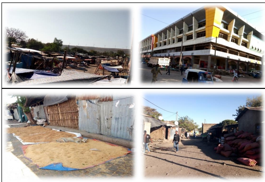
Figure 27: shows the housing regulation and shaping qualities of the place
