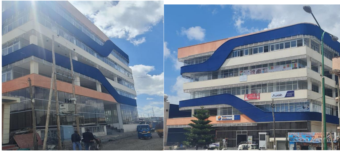
Figure 4.0.7 Awash bank robe mixed use building
