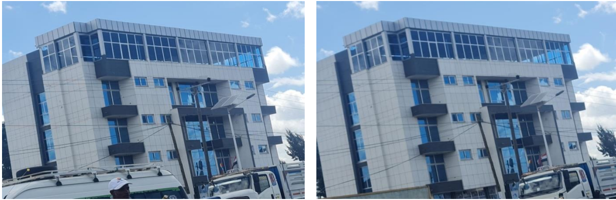
Figure4.0.11 Sena mixed use building.
