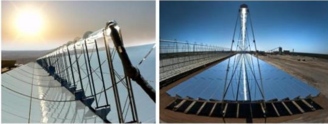
Figure 2.1: Linear concentrating solar technologies; a) Parabolic trough collector b) Linear Fresnel reflector (Lillo et al., 2017)
