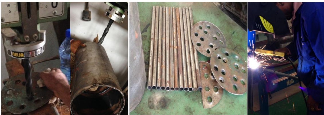
Figure 3.4: Manufacturing of components of EGR cooler
