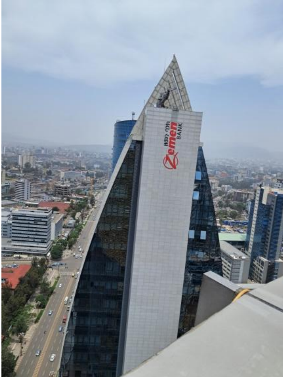
Figure 29 - Zemen Bank Building (Source: Author March 24, 2025)
