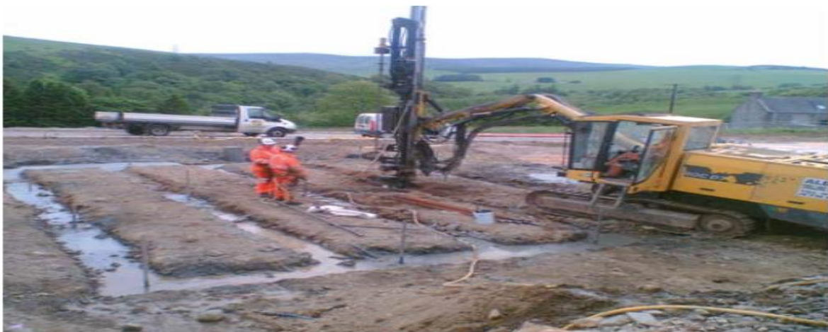
Figure 2-9: Large Track-Mounted Rotary Hydraulic Drill Rig (4)
