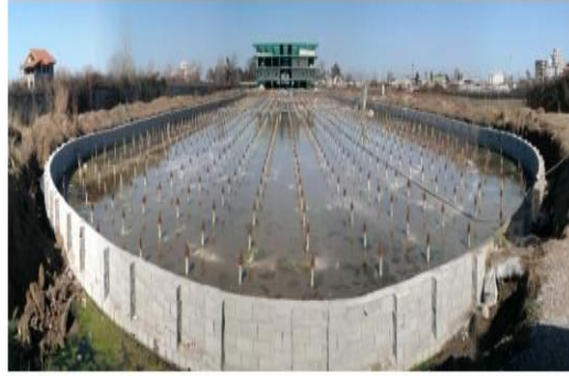
Figure 2-1: Micro piles withstand axial and/or lateral loads. (Iran, Mahmoudabad, Narenjestan-Southern site) (34).
