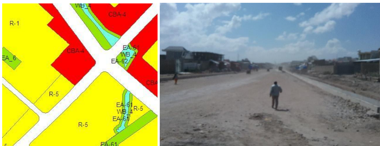
Figure 22: A 30 m road is being built according to the plan
