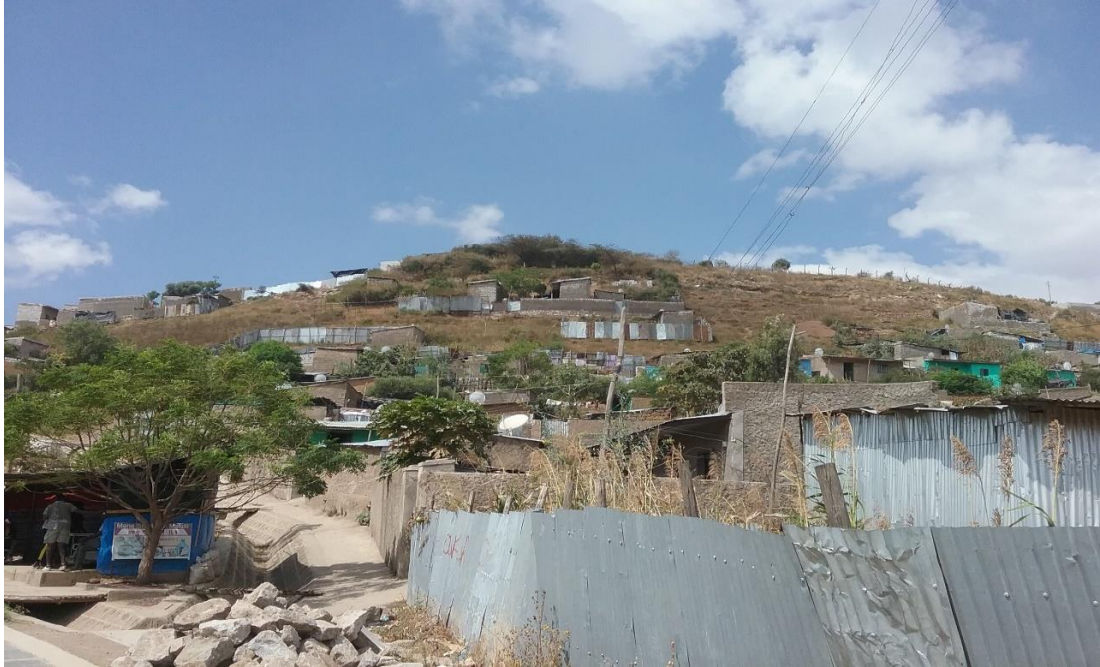
Figure 12: increase of illegal houses has contributed to the extent of the structural plan of Adama city
