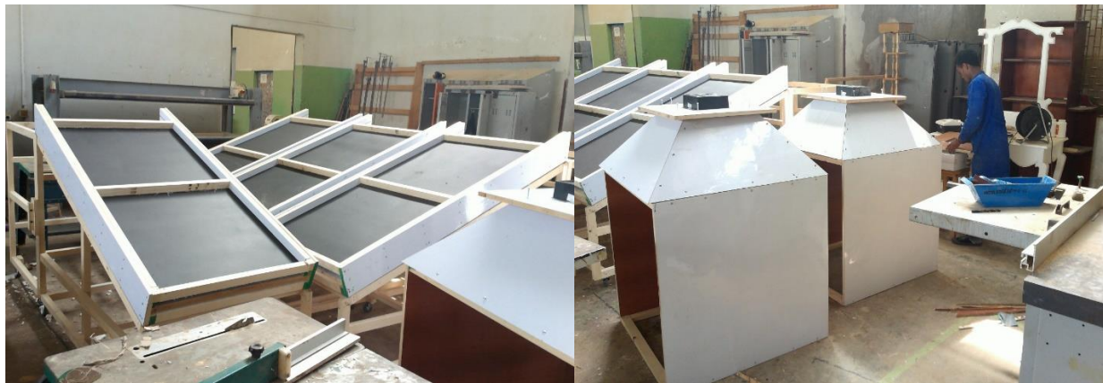
a) Collector and drying chamber construction
