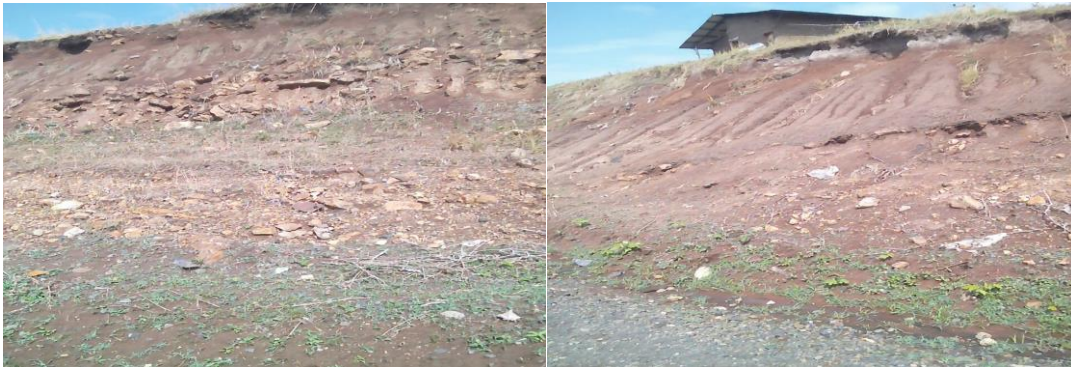
Figure 4.7 Residual soil in the study area
