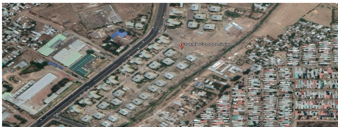
Figure 4:2: Duket condominium site (Source: google earth)
