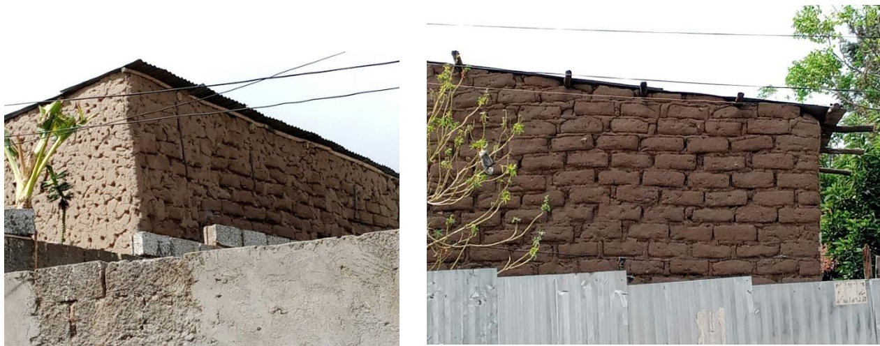
Figure 15. Mud block construction for external walls
