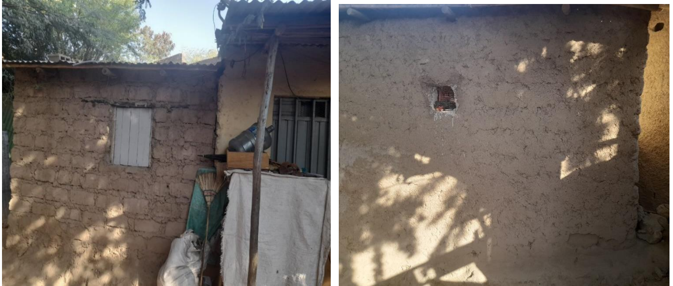
Figure 16. Narrow window opening
