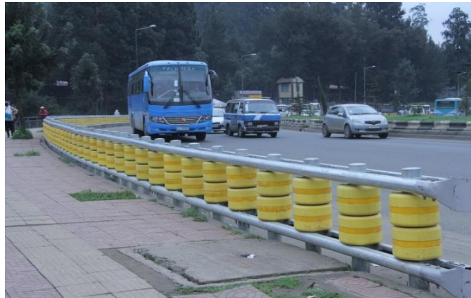
Figure 2. 20: Roller type roadside-crash barrier (Ethiopian transport bureau report, 2021)
