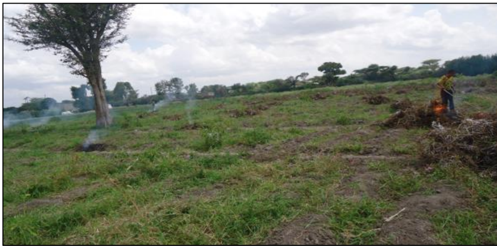
Figure 4. 5 Different weed and unwanted material removal before land preparation
