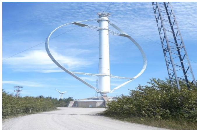
Figure 2.2 Vertical axis wind turbine (VAWT) (ChristianT, 2010)
