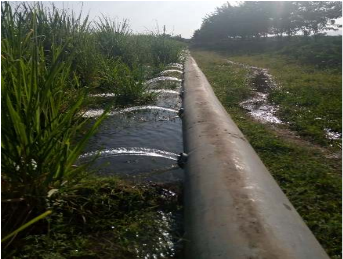
Appendix figure 2: Hydro flumes irrigation method in kesem Sugar Project
