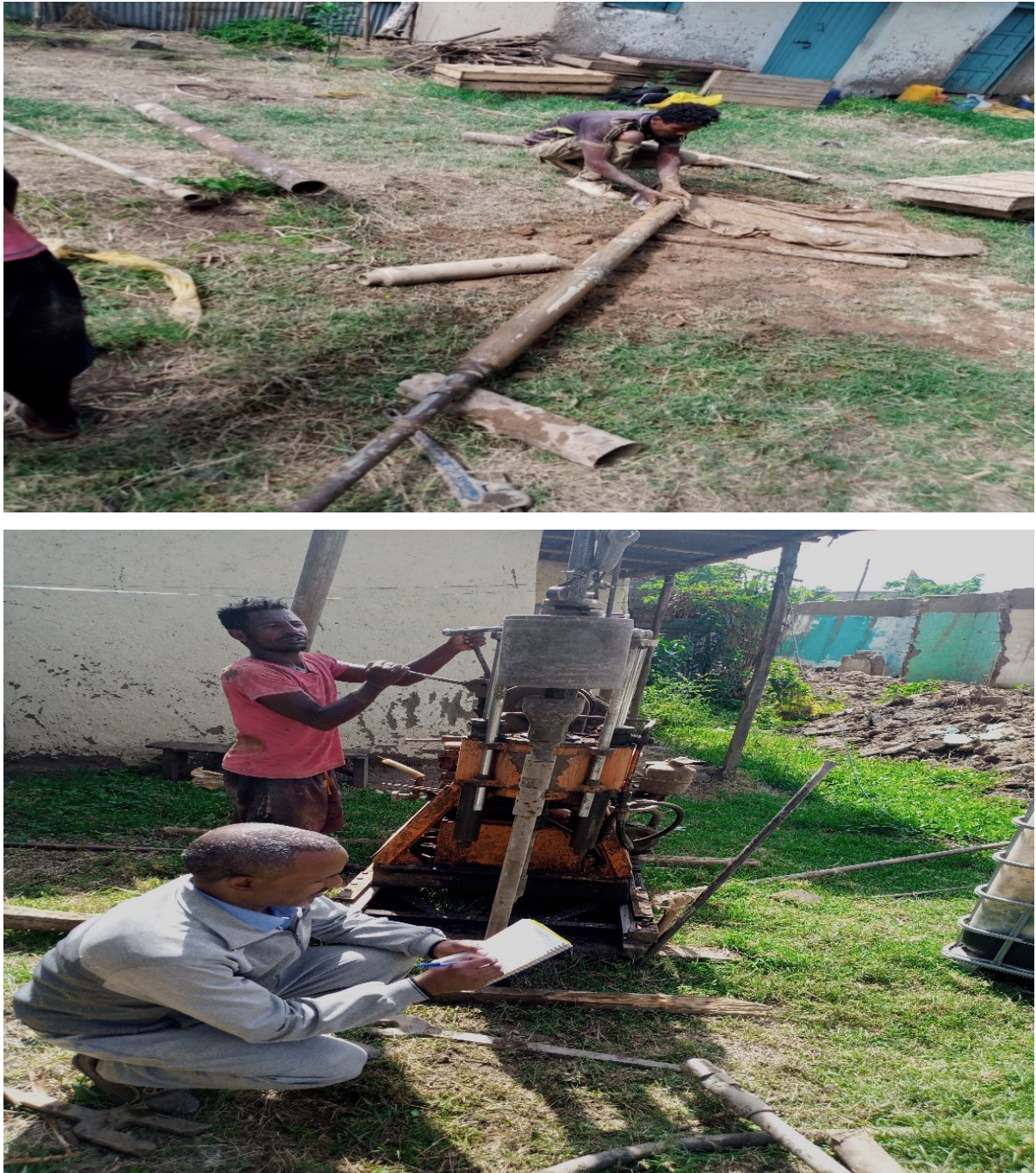
FIGURE 3.2 Partial View of the Project Site
