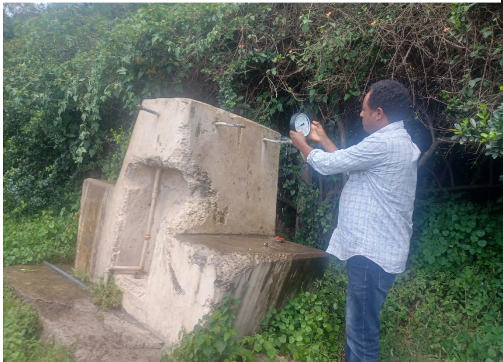
Picture 1: Field pressure measurement
