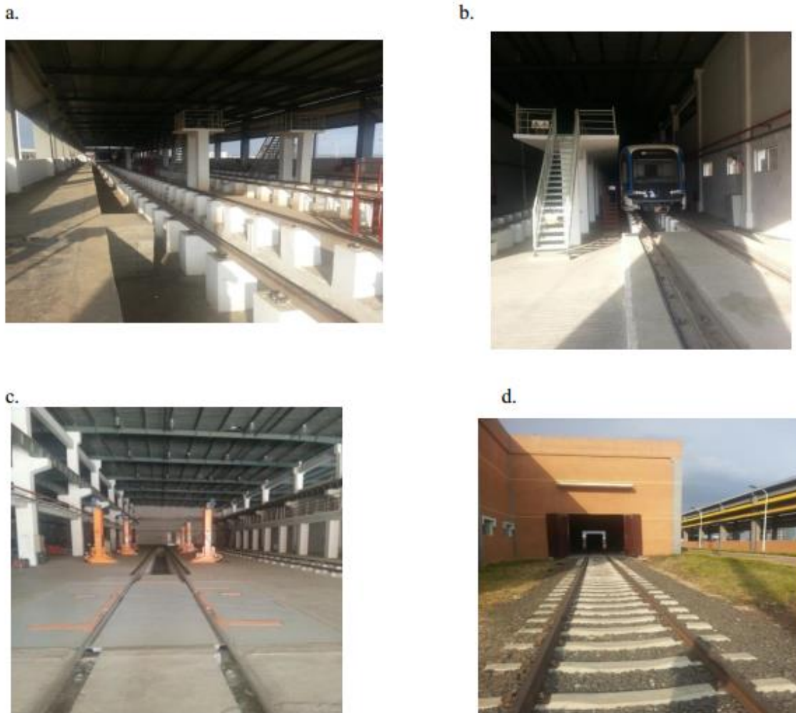
Figure 3. 1 a) daily inspection workshop b), monthly inspection workshop
